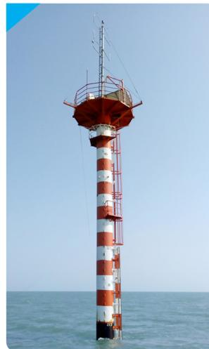
Deployment of buoy for offshore data collection using surface buoy with a deep-water mooring to obtain hourly data. Installation of offshore data collection platform at Gulf of Khambhat and Gulf of Kutch, for wind profile measurements.
