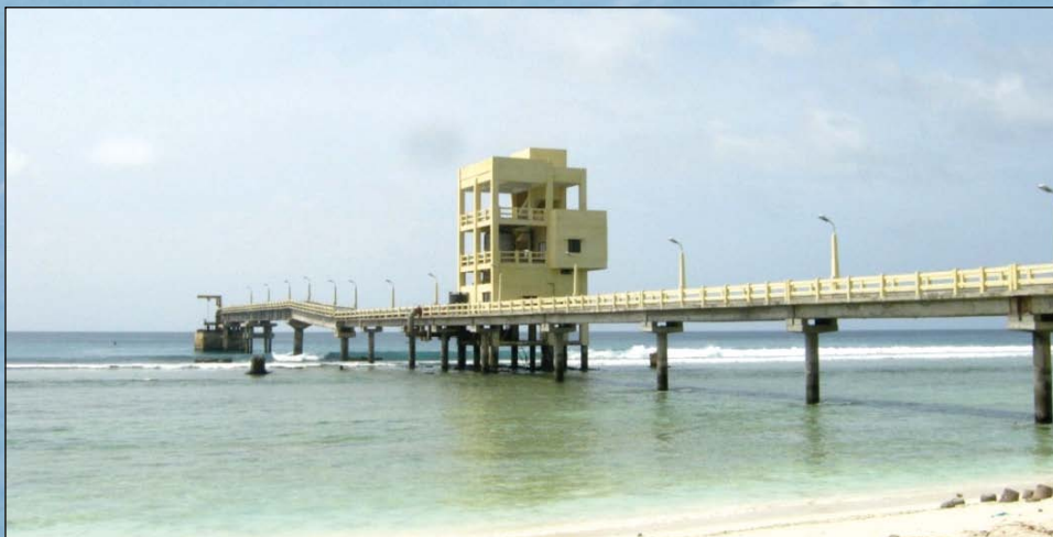
Desalination Plant, Agatti UT Lakshadweep
