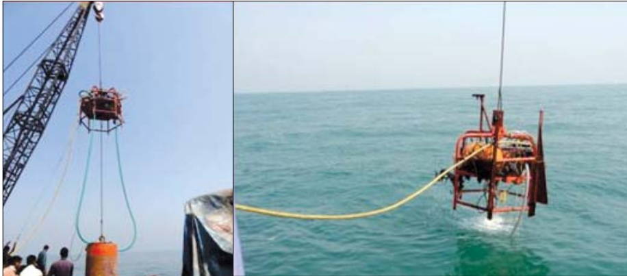
Suction Pile Demonstration
