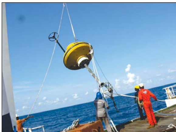
Tsunami Buoy Deployment
